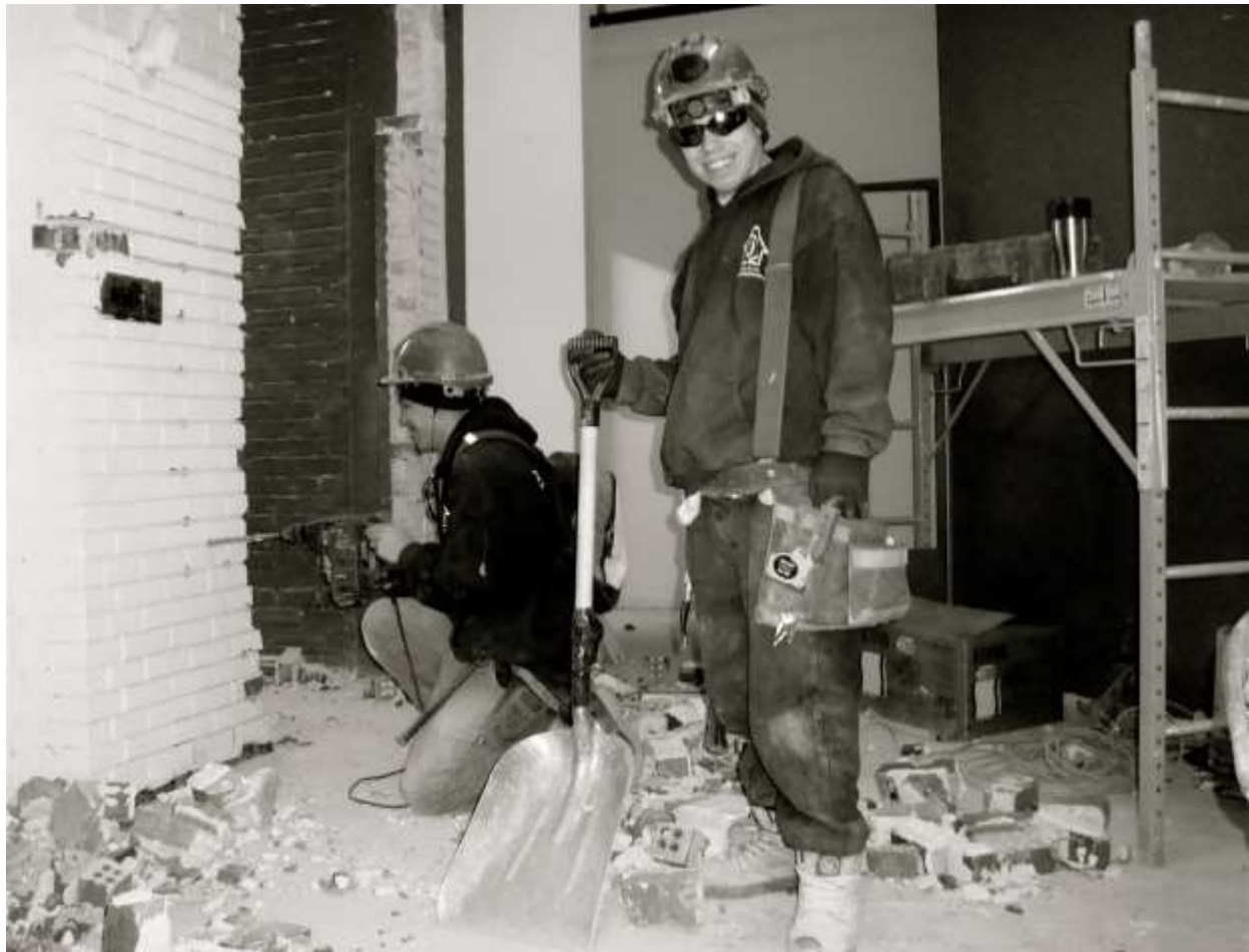
Breaking through walls: Two BUILD Apprentices Dillon (front) and Jordan (back) making a new entryway to the second-floor of the SEC. The renovation included adding a new stairwell on the east end of the building.
